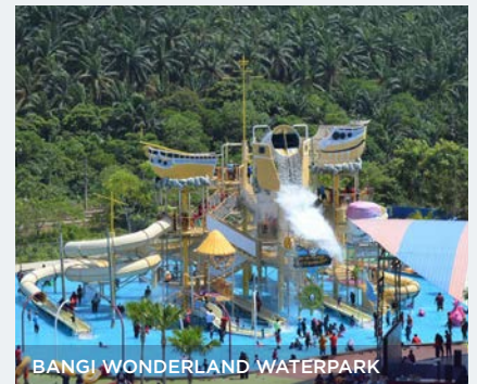
BANGI WONDERLAND WATERPARK Client Bangi Wonderland Location Kajang, Malaysia Area 5.000 m 2 Construction Date 2020
