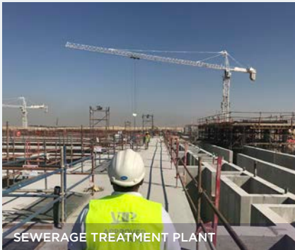
SEWERAGE TREATMENT PLANT
